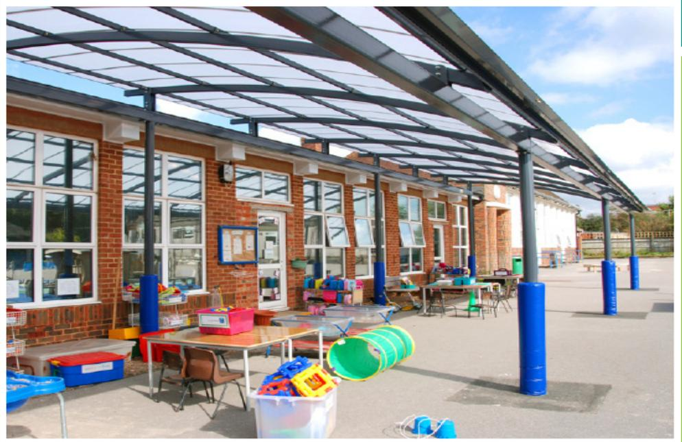
The 16mm triple clip polycarbonate system is used to create a hard wearing roof covering for our canopies.
